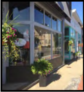
2.a.i. Storefronts and large display windows are inviting and provide visual interest and depth to the district.
